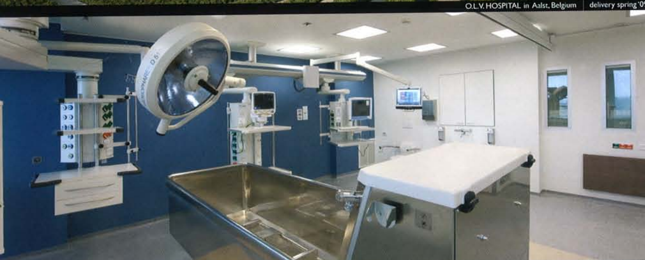
MILITARY HOSPITAL in Brussels, Belgium | European Reference Center for Burns treatment | delivery autumn '09
