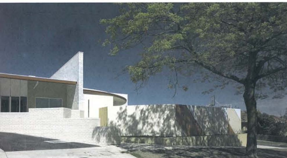
Box Hill Adolescent Mental Health Unit was designed with curved roofs, cream block work and large expanses of glazing
